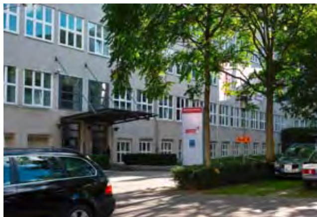
Bürocampus Wangen, Stuttgart-Wangen
